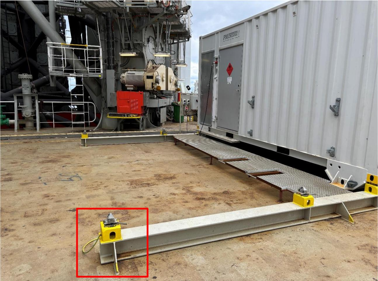
**Figure 8-2 – Grounded connections of 20ft container**
