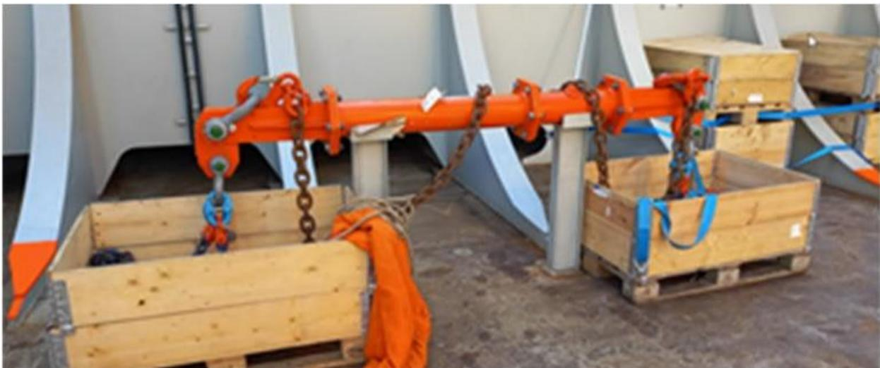
**Figure 8-3 – Seafastening of the lifting frame example**
