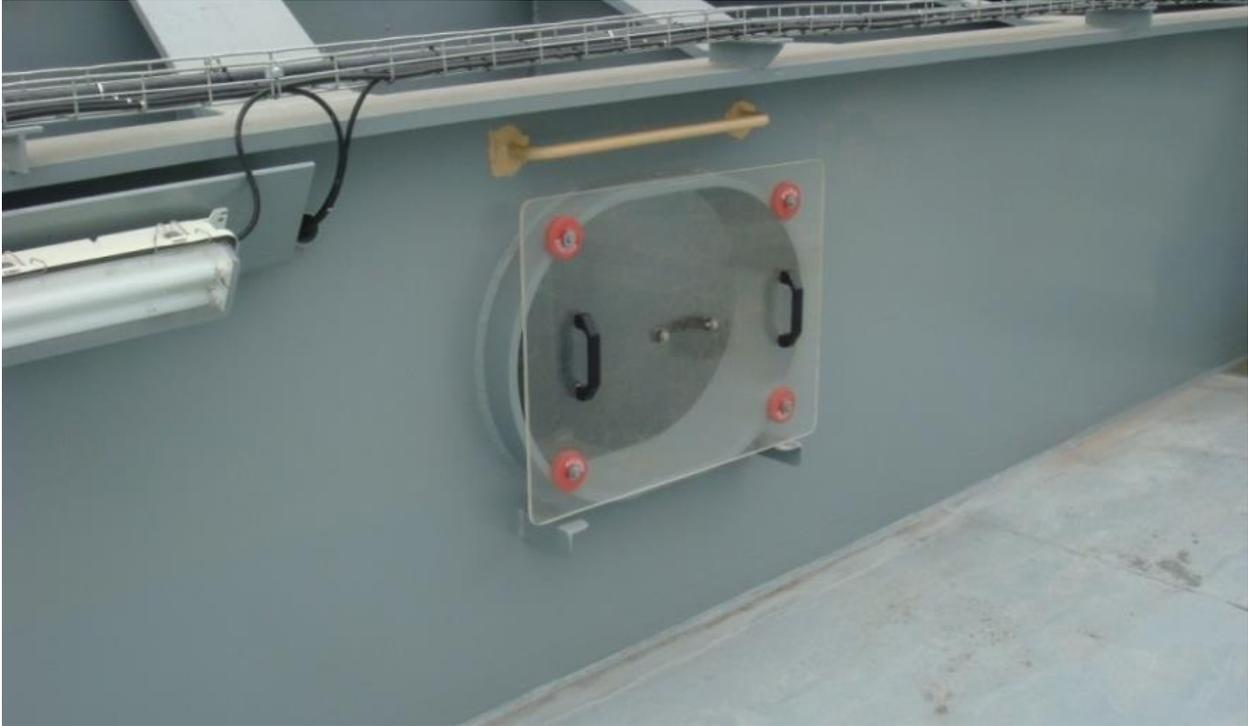
**Figure 4-3 – Sealed access manhole and water drainage example**
