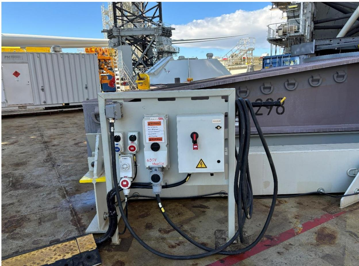
Figure 5-9 - Nacelle frame seafastening power supply example
