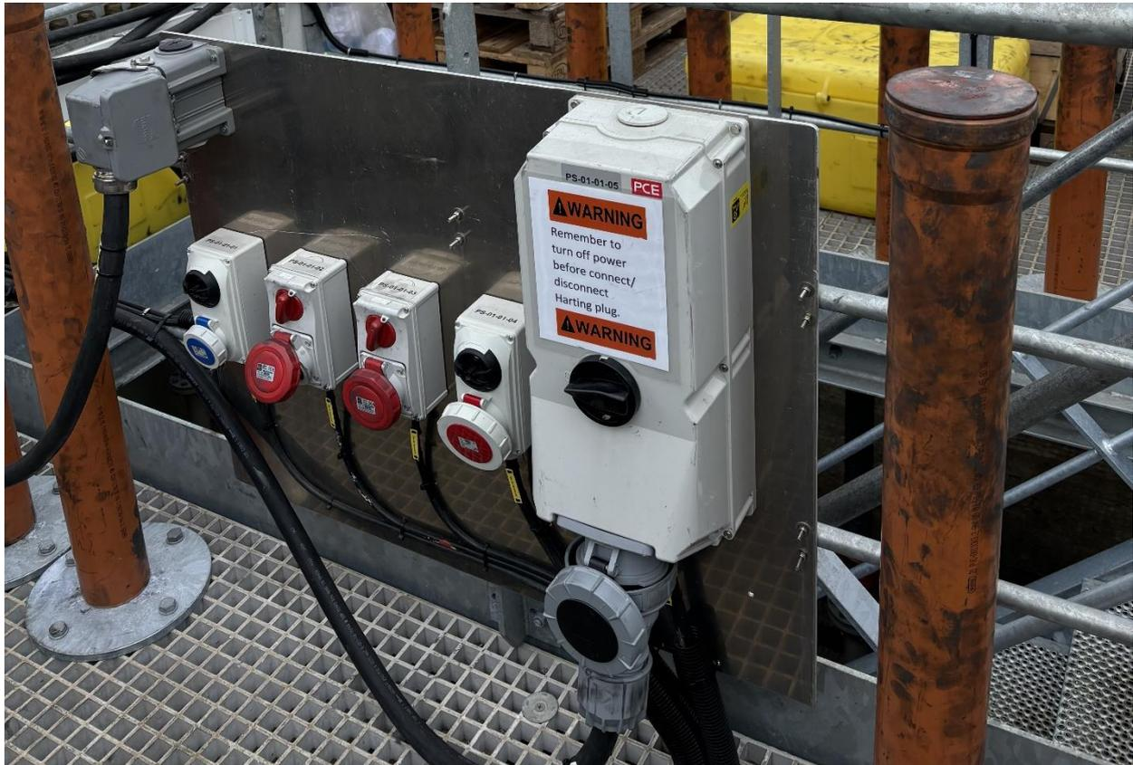
Figure 4-12 – Tower seafastening light and power outlets example
