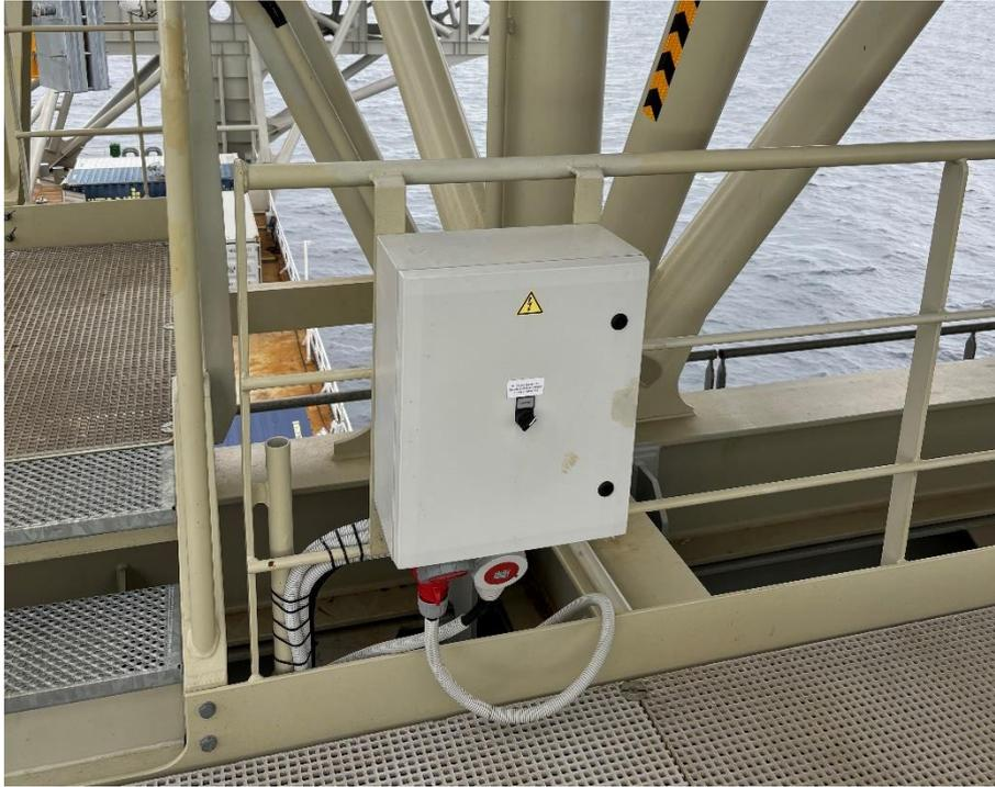
**Figure 6-15 - Power Supply on blade rack example**
