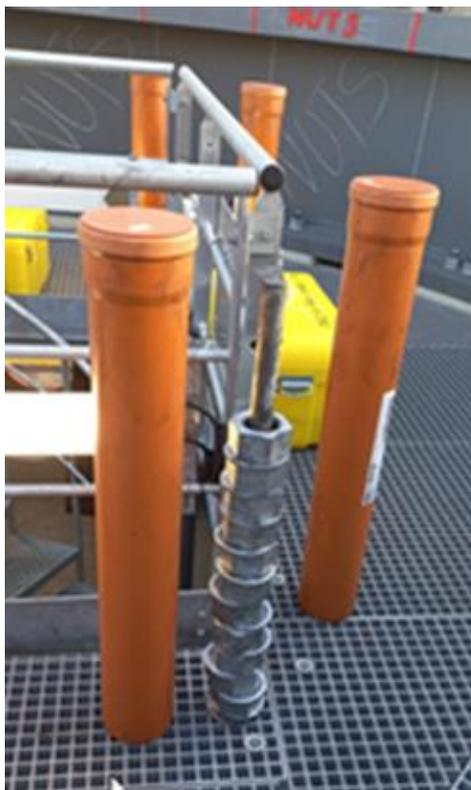
Figure 4-11 - Storage solution for nut and washers in the tower grillage example
